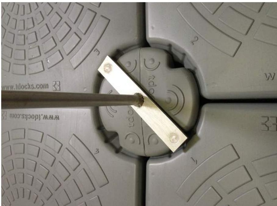
8. Now you need to lock together all the lugs around the outside. N.B. before locking lugs 1 & 4 together (this should be the side facing the shore) you will first need two spacers (SKU 3145) to fill the gap between the lugs.
